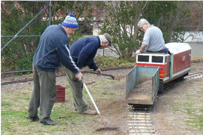
The track crew at work
