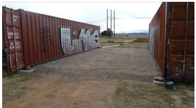
Floor of Workshop being prepared for concreting.
