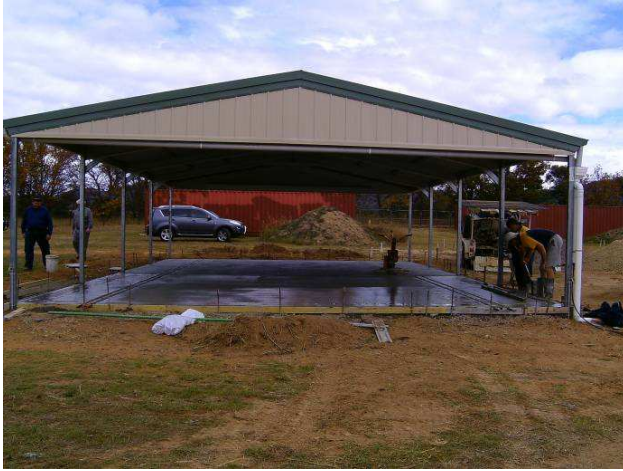
Completed station floor
