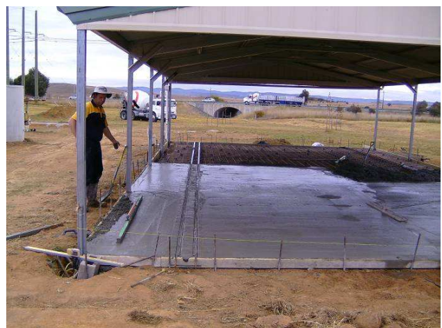
Station floor being poured
